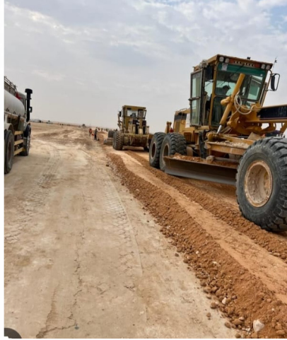
Backfilling And Compaction
