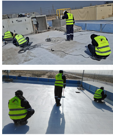
Waterproofing & Concrete Repair
